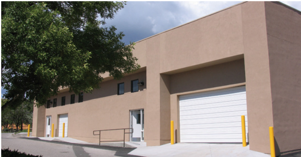
New maintenance building, University of New Mexico
